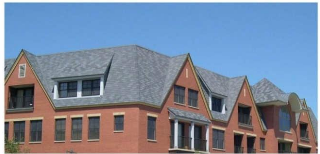
Roof Materials: Asphalt Composite Shingles
